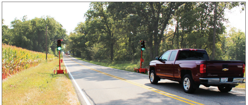
Pictured above is a Rock Energy work zone along Highway 67 in Clinton, WI. New portable stop lights at the work zone sense incoming vehicles from both directions and automatically change accordingly, allowing for vehicles to pass through the one-lane work zone safely.
