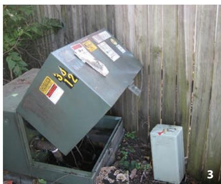
1. This transformer is almost entirely covered with vegetation that prevents lineworkers from accessing it for repairs and routine maintenance. 2. This bush grew too close to the transformer. Remember to plan for a plant's growth when landscaping. 3. This fence was built so close to the transformer that the hinged box cannot be opened. Workers need at least 10 feet of clearance in front of the box and 4 feet on the other sides. 4. Debris like this around a transformer is a safety hazard.
