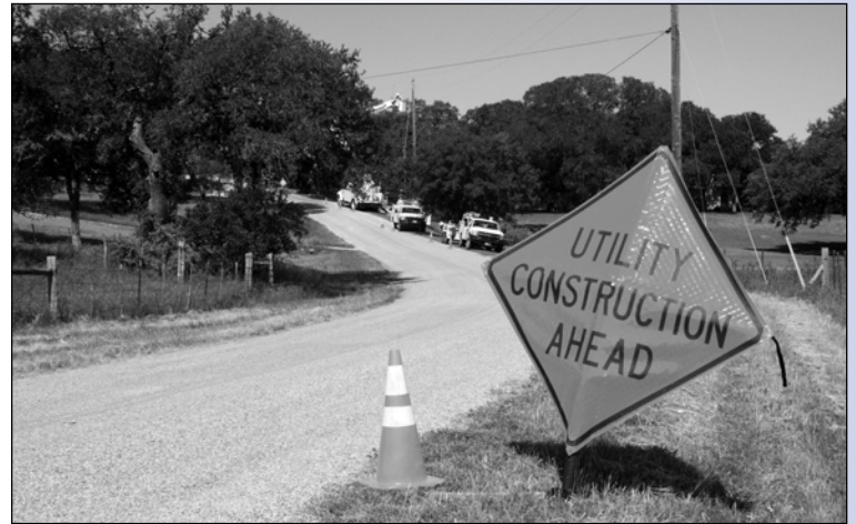
Warning signs, orange cones, and flashing lights all indicate a work zone on the road ahead.
