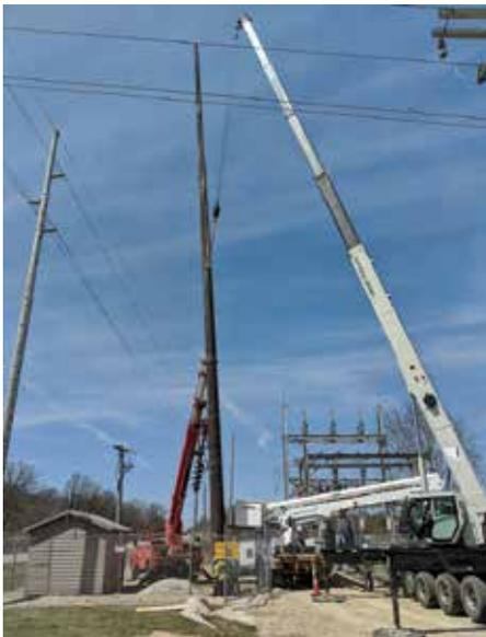
This pole being set at the Orfordville Substation is one of 12 new poles needed for the new AMI system. The 110-foot poles are placed 13 feet into the ground and stand 97 feet above ground.
