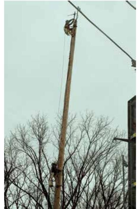
A worker mounts an antenna at the top of a 70-foot existing pole at the Shaw Substation. The antennas, which are placed strategically throughout our service territory, will transmit meter information to the co-op via a licensed, encrypted, secure system.
