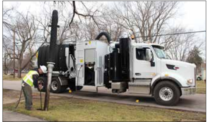
J&R Underground is working with Rock Energy on the projects. Its vacuum excavation truck is used to locate existing facilities. This work must be done before the upgrade begins.
