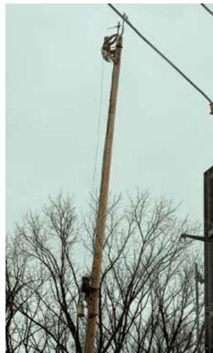
A worker mounts an antenna at the top of a 70-foot existing pole at the Shaw Substation. The antennas, which are placed strategically throughout our service territory, will transmit meter information to the co-op via a licensed, encrypted, secure system.
