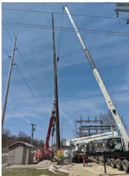
This pole being set at the Orfordville Substation is one of 12 new poles needed for the new AMI system. The 110-foot poles are placed 13 feet into the ground and stand 97 feet above ground.
