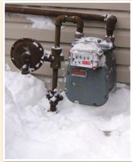
As you're shoveling sidewalks and driveways this winter, remember to check your natural gas meter and pipes for drifted snow, top, which can cause problems. When exposing the meter and pipes, avoid using a snow blower. Instead, gently remove snow and ice from the area. Also remember to clear snow away from furnace intake and exhaust pipes.
