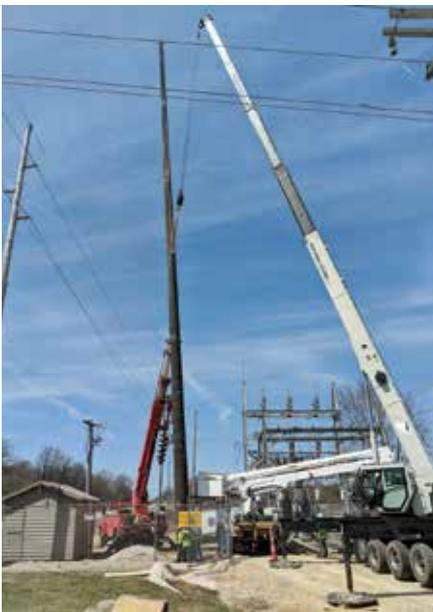
This pole being set at the Orfordville Substation is one of 12 new poles needed for the new AMI system. The 110-foot poles are placed 13 feet into the ground and stand 97 feet above ground.
