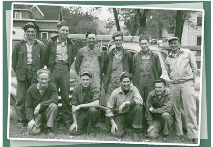
Rock County Electric Cooperative's line crew in charge of construction and maintenance in the early 1940s was, from left, front: Ed West, Lavern Brecklin, Leroy Fitzsimmons, Mervin Stone; back: Al Manthey, Don Williams, James Polglaze, Kenneth Hessenauer, Hugh Curtis, and Line Superintendent Phil Yuengst.
